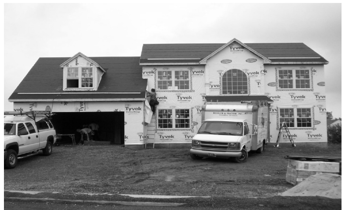
Bethel Township $276,900 UNDER CONSTRUCTION
